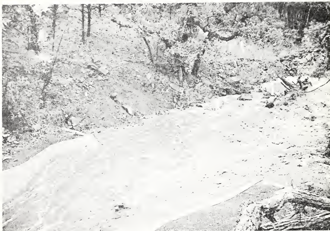
Figure W-16. --Here is the flume in high water. One minute after this picture was taken the treetop had passed through the flume. The top was 24 feet long and 28 inches in diameter.
